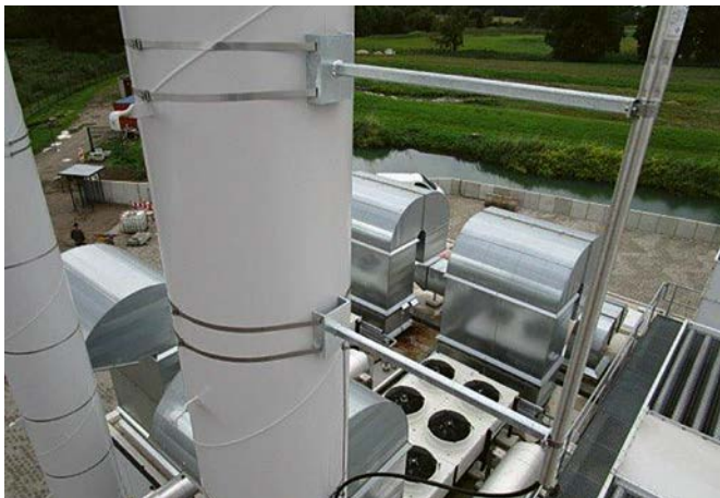
Spacer with tensioning strap fastener
